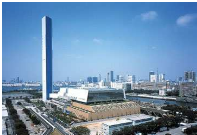
Chuo Incineration Plant, Tóquio (Foto Hitachi)
